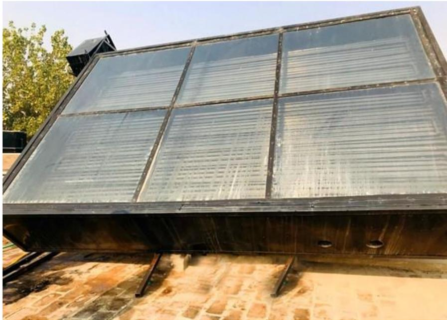
**Figure 1: The Flat Plate Solar Collector Assembly**
