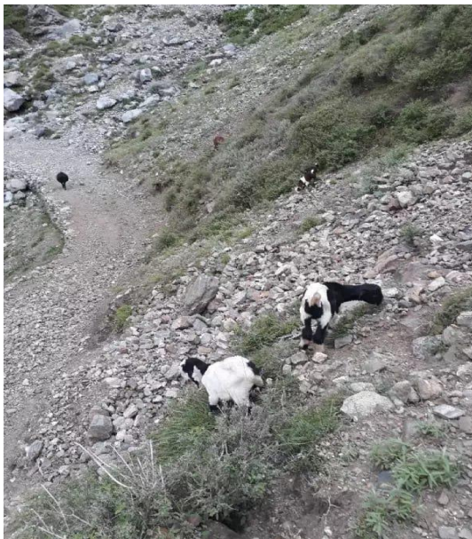
Figure 9: Land sliding causes erosion
